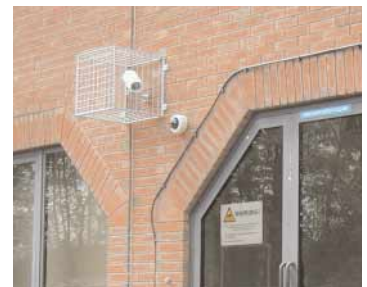
Vandal resistant camera monitoring a security entrance, together with a Siemens outdoor PIR
